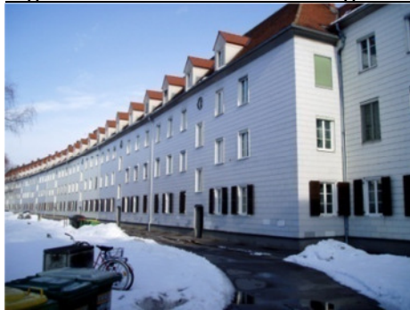
Figure 4 Residential buildings Graz, Dieselweg, situation in 2008 before renovation
