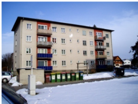
Dieselweg 4,6,8 (year of construction 1958)
