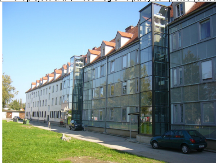
Figure 6 Refurbishment project Graz, Dieselweg 3-19 partly completed (October 2009)
