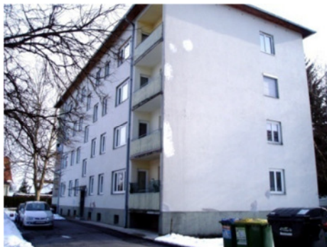
Dieselweg 12, 14 (year of construction 1968)
