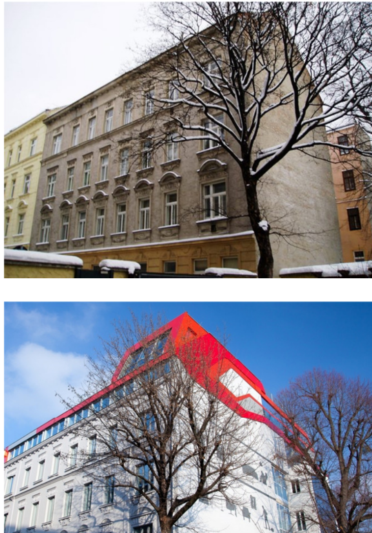
Figure X.8 Residential building Vienna, Wissgrillgasse, before and after major renovation
