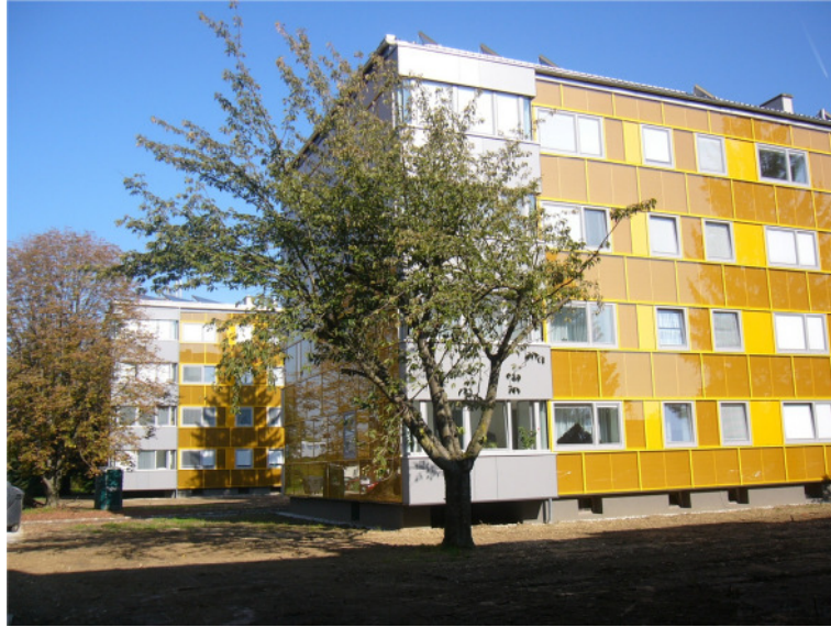
Figure 7 Refurbishment project Graz, Dieselweg 12 and 14 with solar thermal collectors already installed (October 2009)
